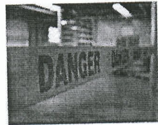
Caution warning tape
